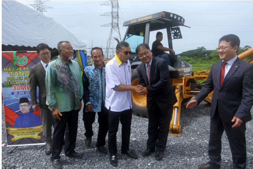
LAUNCHING: Azlan Man (fourth, left) shakes hands with James Lee (second, right) at the Groundbreaking Ceremony of the 30MW Large Scale Solar Project in Chuping yesterday. — Named Pictures
